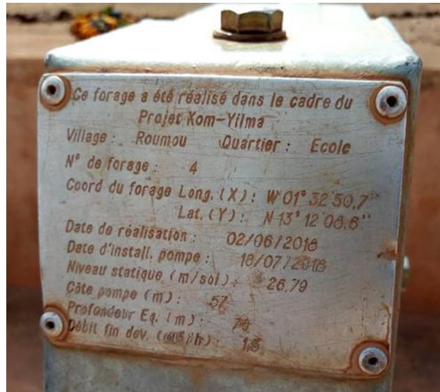
Figure 16: Example of water point identification plate
